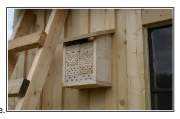
From top to bottom the hole sizes are 2,4,6,8 and 10mm The actual positions and locations don't need to be precise.
